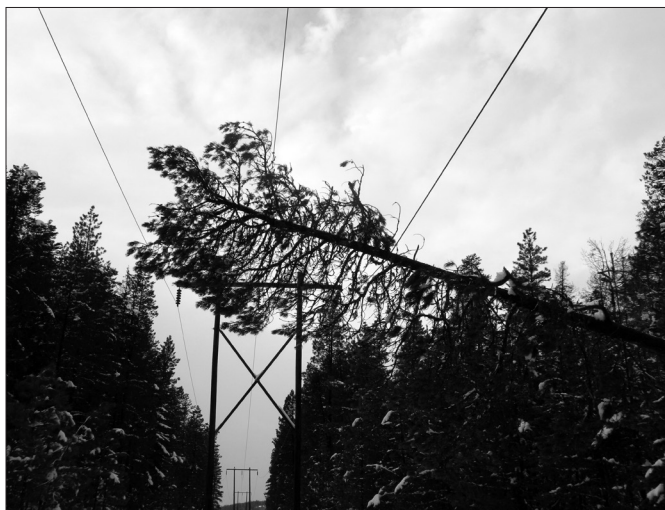
Lineworkers for Klickitat PUD untangled trees from the utility's Glenwood transmission lines after snow and ice in January 2012 brought down limbs and trees.
